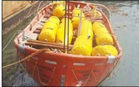
Using water bags during load test 141
