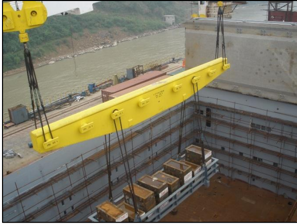
Load testing for twin crane operation
