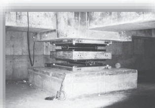
Fig. 9 Simple roller bearing [10]
